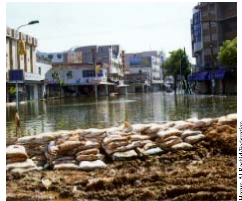
Dykes along rivers and waterways in south and central China provide relief - often only temporary. By June 1999 more than 6,200 km of dykes had been reinforced.
