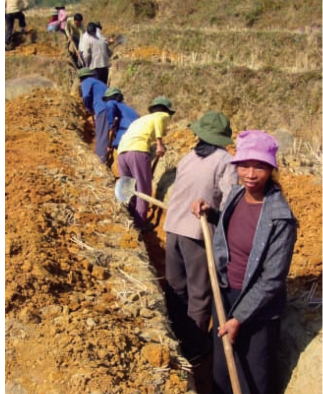
Local villagers prepare the way for the new water supply system.
