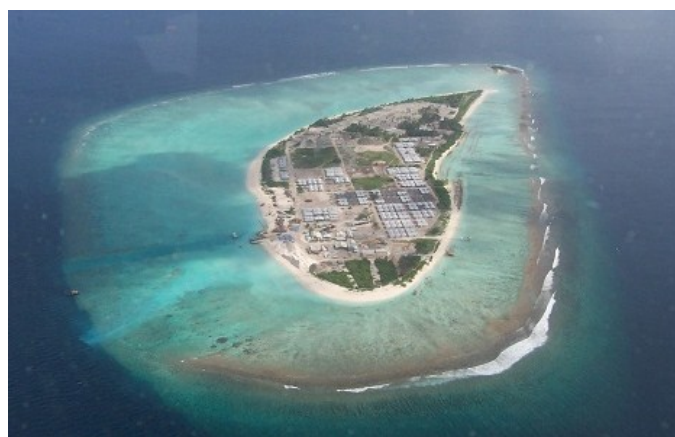
Following the impact of the 2004 Indian Ocean Tsunami on the Maldives, the Red Cross constructed an entirely new settlement on the Island of Dhuvaafaru. Homes and infrastructure were constructed for over 400 families who were relocated from a neighbouring island which was badly affected by the tsunami because the protective coral reef surrounding the island had been largely destroyed.
