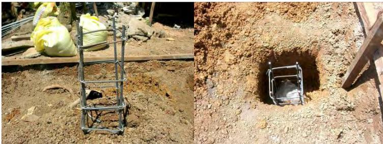
Within the foundations of the new houses, typhoon –resistant building techniques such as embedded scaffolding will help hold up structures in the face of strong winds and storms. Previous makeshift homes had no such advantages and it was necessary to rebuild homes every year. (Photos: International Federation of Red Cross and Red Crescent Societies)
