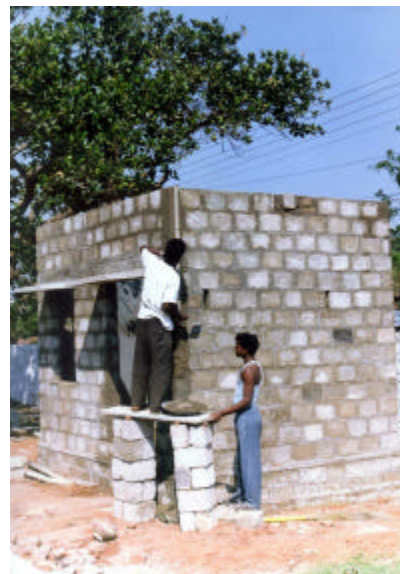
Finalising the work on a cyclone-resistant house.
