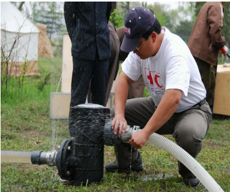
International Federation water and sanitation officer, Mr. Kim Song Il, assembles an emergency water and sanitation unit during training in Anju City, South Pyongan Province, April 2008. Terje Lysholm/International Federation.
