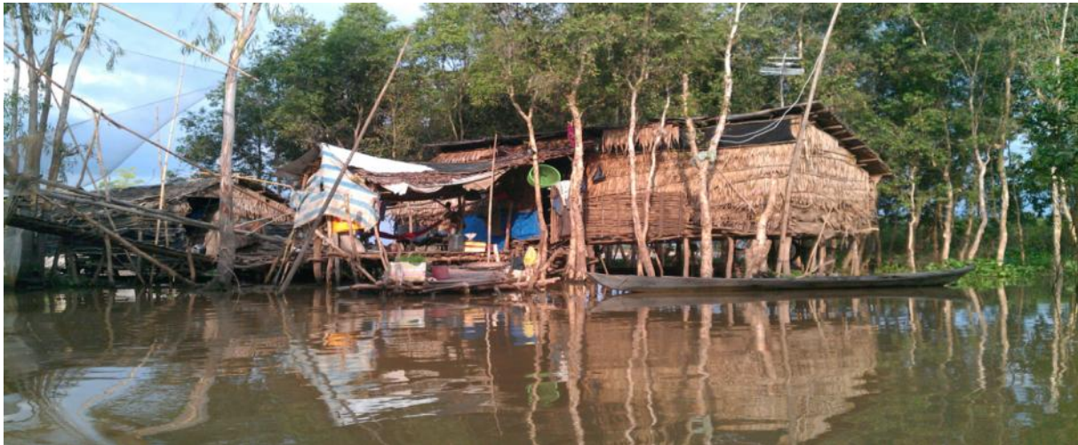
Moc Hoa district, Long An province: Houses like these are common across the Mekong region in south Viet Nam. During the floods, inhabitants raise their homes to save them from being swept away by floodwaters. (Photo: DWF)
