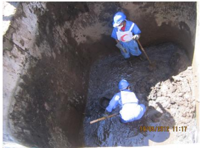
Comoros Red Crescent Society volunteers cleaning affected water tanks in the most affected villages. May 2012. Photo/ CRCO
