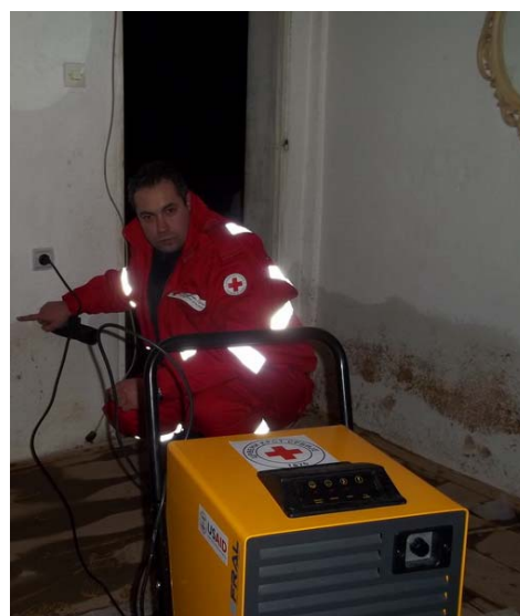
Red Cross of Serbia National Mobile Technical Team member is dehumidifying the flooded home on 27 th February. Photo: Red Cross of Serbia
