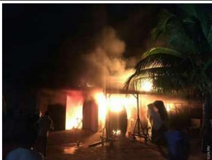
The fire at the power house of Gdh. Thinadhoo on 26 January at 2:30. The power house was destroyed beyond use during the fire. Photo: SunMV
