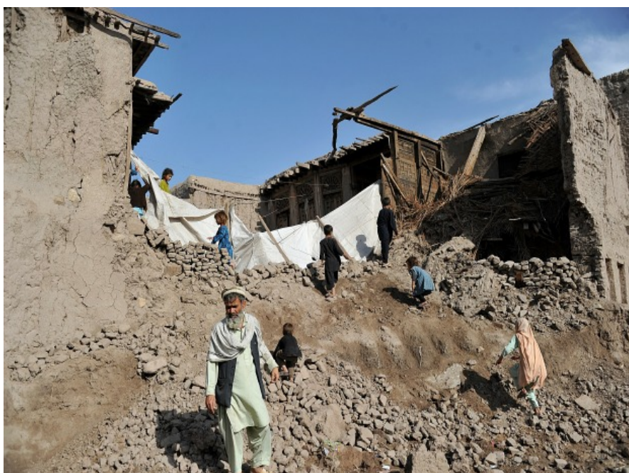
One of the many houses damaged by the 24 April earthquake in Kunar province, eastern Afghanistan. Photo credit: afpak.foreignpolicy.com
