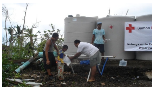
SRCS water sanitation coordinator is explaining to the beneficiaries how to use jerry cans to collect clean and chlorinated water produced by the NOMAD system stored in these tanks. Photo credit: SRCS
