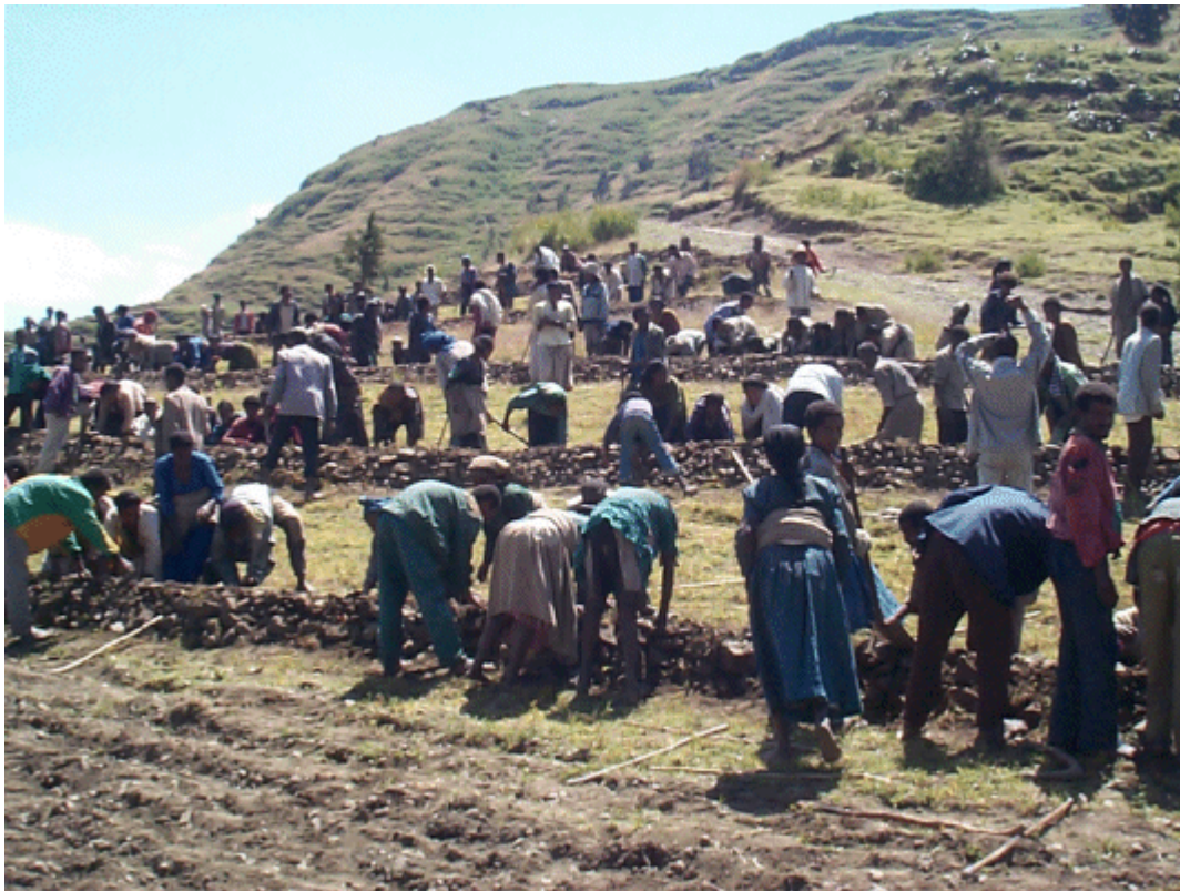
Terracing project in South Wollo
