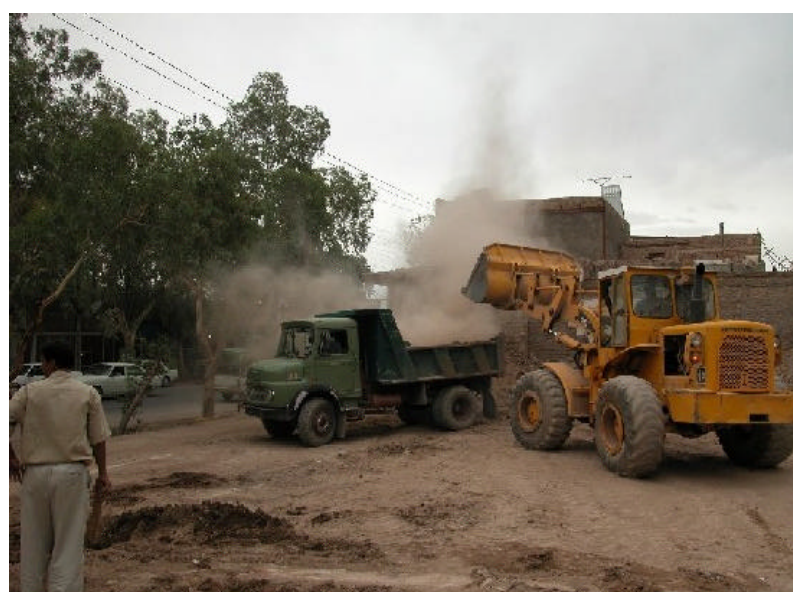
Cleaning of the construction site for the Urban Health Centre
