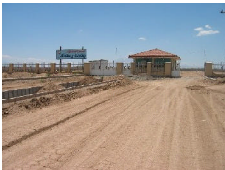
The general view of the Road Rescue Base construction site
