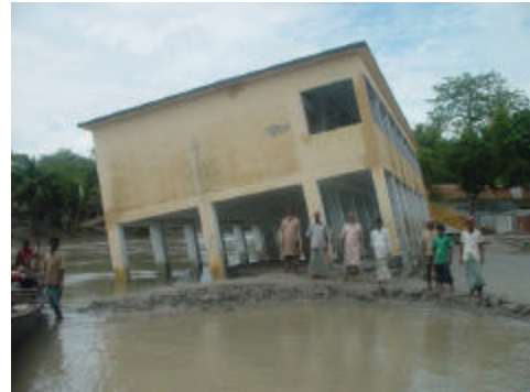
Washed away school building in Sirajganj
