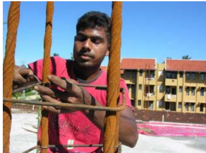
Construction of Janaraja school by the Irish Red Cross in Kalutara
