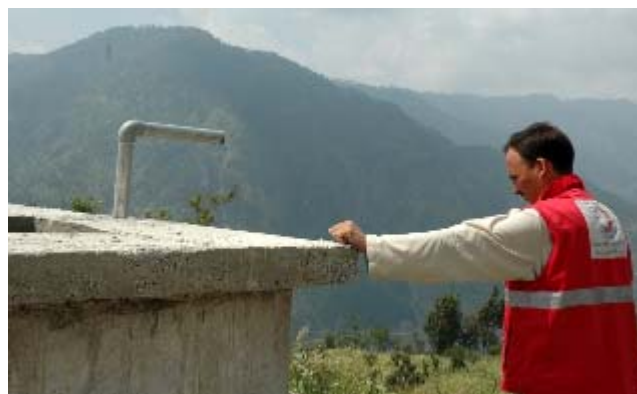
This 17,000 litre water tank constructed by the PRCS services 120 families in the remote village of Gali Chaparran high in the hills above Balakot. (Photo: IFRC)
