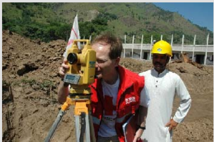
A construction delegate checking progress at a degree college in Pakistan-administered Kashmir. (Photo: IFRC)
