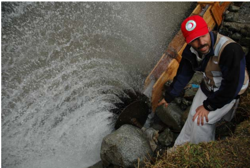
PRCS livelihoods programme officer inspecting a hydropower generator constructed by PRCS/International Federation at village Kushgram in Allai Valley. The generator runs on the kinetic energy of water and can produce five KVA electricity. Now 130 households in this remote village of northern Pakistan have access to electricity. Photo: Mubashir Fida/ International Federation.
