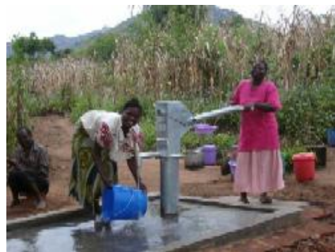
The successful rehabilitation of this borehole hand-pump has provided clean water for these women in Zomba district, Malawi.
