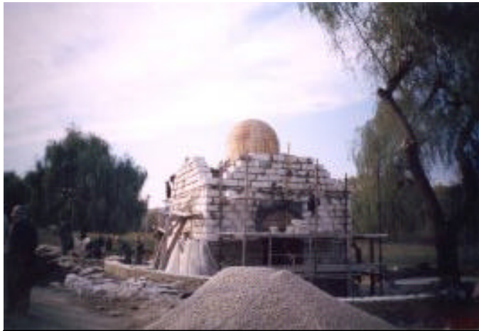
Nearly-completed well reconstruction in Curchi, Orhei district
