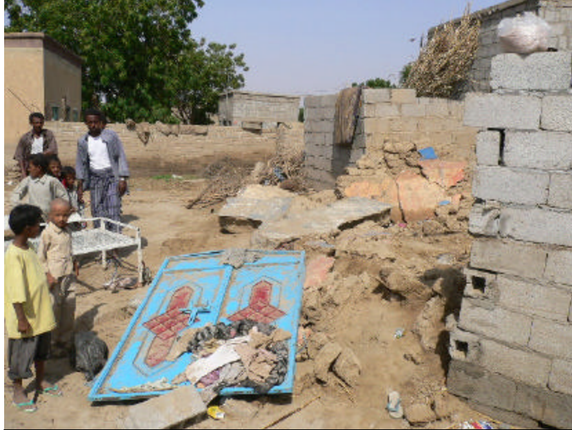
Devastating: even solid structures failed to withstand the floods.
