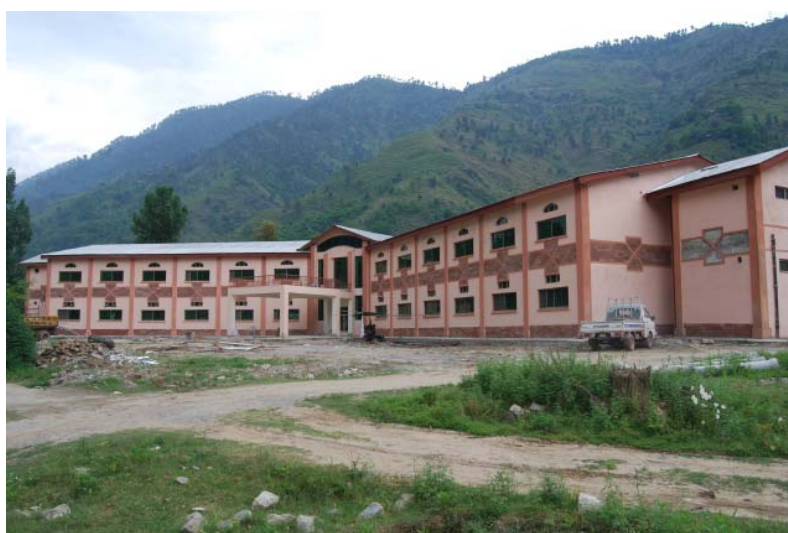
The newly constructed boys' degree college in Garhi Dupatta (Pakistan-administered Kashmir). Photo: International Federation.
