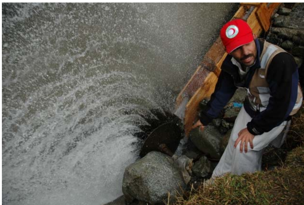
A Pakistan Red Crescent Society livelihoods programme officer inspecting a hydropower generator constructed by Pakistan Red Crescent Society/International Federation at Kushgram village in Allai Valley. The generator runs on the kinetic energy of water and can produce five KVA electricity. Now, 130 households in this remote village of northern Pakistan have access to electricity. Photo: International Federation.
