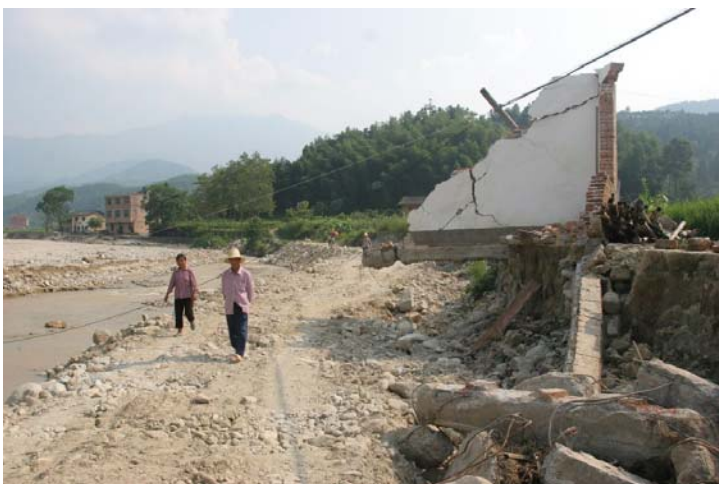
A couple walking along one of the destroyed buildings.
