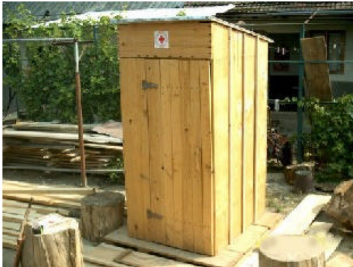
Latrine construction in Rast camp in Dolj county
