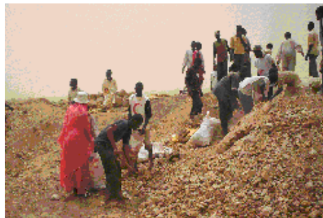
SRCS volunteers filling sand sacks for strengthening river banks in Khartoum.
