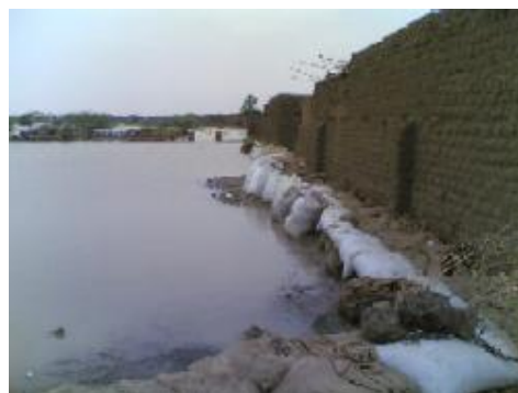
Rivers burst their banks and floodwaters destroyed agricultural land as well as property, including many houses.
