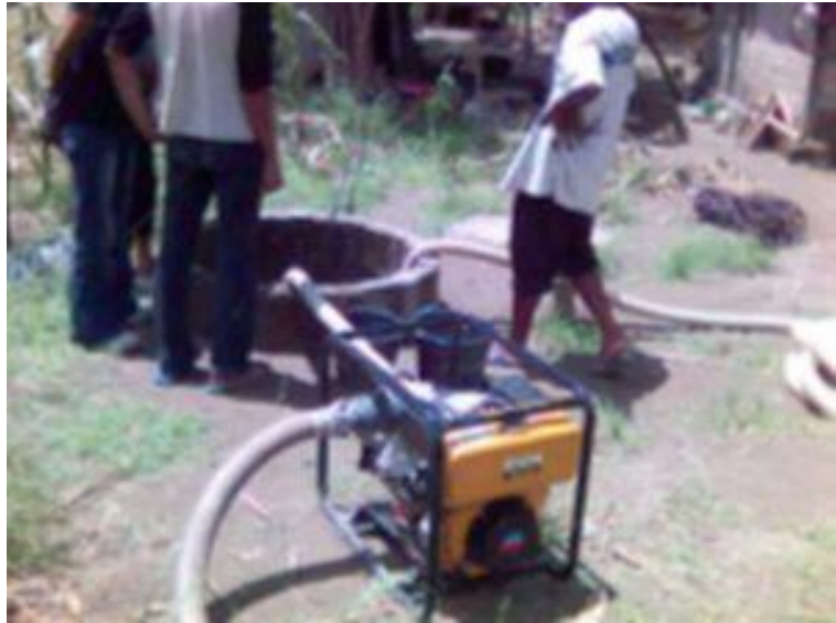
Treated deep wells restore clean and safe water to affected communities.
