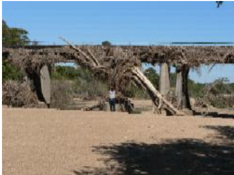
The aftermath of the floods at the Railway Bridge along the Ngwezi River.
