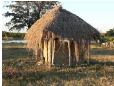
A makeshift pit latrine at Kasaya Basic School; in the background is a dam which is the source of water for the community.
