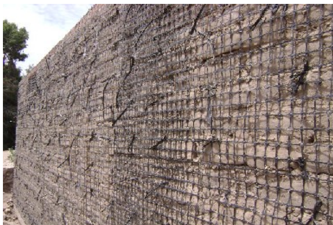
The International Federation and the Pontificia Universidad de Católica del Perú (PUCP) will use reinforced adobe with geogrids ( geomalla ), similar to technique shown in the picture at the left, in the earthquake-resistant houses to be built in the Cabeza de Toro community in Independencia district in Pisco. Source: International Federation
