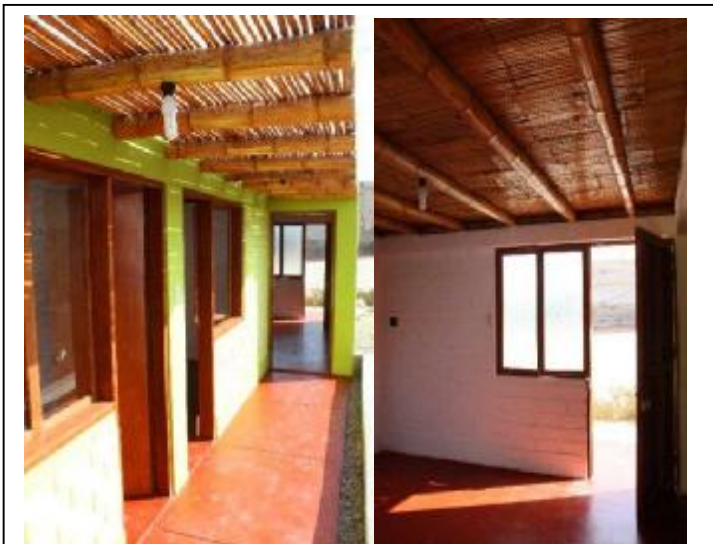
Houses built by the International Federation and its partners, like this one in San Clemente (Pisco), provide better quality of life to the target population. International Federation / J. Ormeño
