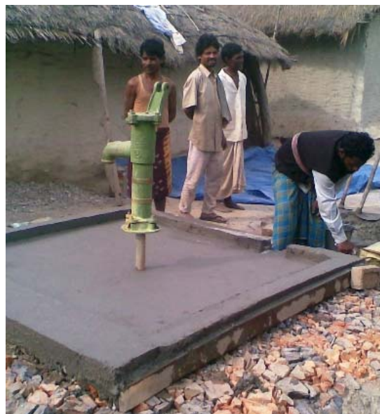
A tube well being renovated in Sarlahi district.
