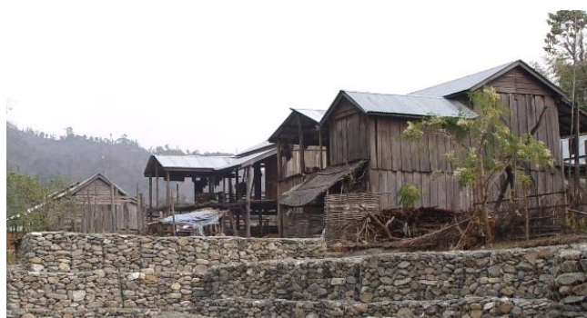
Houses made safe in Udaypur district with retention walls.
