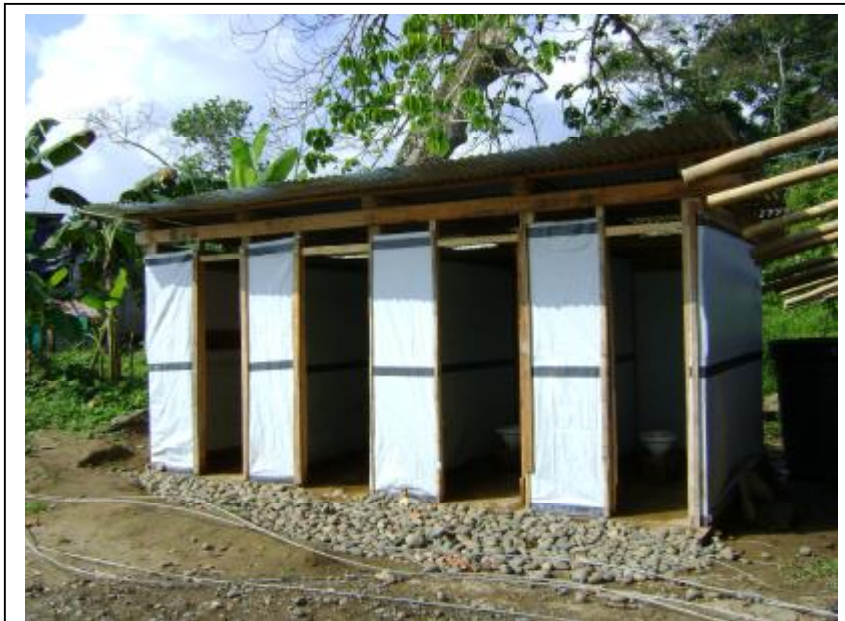
Latrines constructed in the community of Miras Palmas. Source: International Federation/ C. Ferrer
