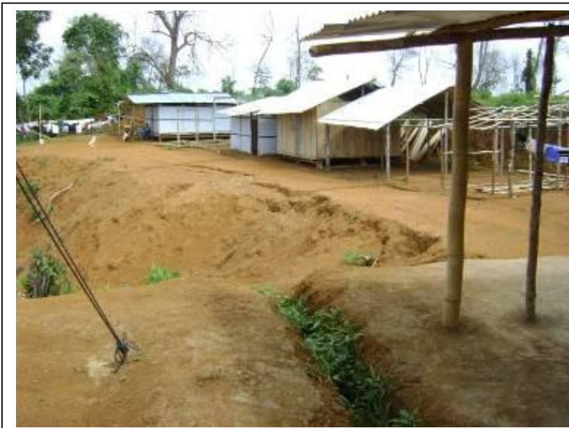
Shelter kits were used to improve these homes in the community of Achotal. Source: International Federation
