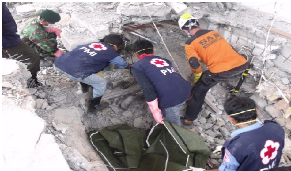
Indonesia Red Cross (Palang Merah Indonesia/PMI) volunteers digging through rubble to look for survivors in Padang. Photo: Wayne Ulrich/International Federation.
