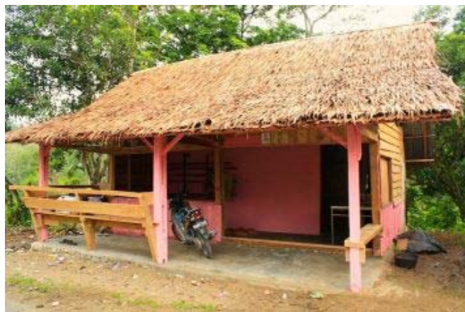
A completed rumah tumbuh in Sungai Lundang, Pesisir Selatan District. The owner has painted the shelter pink and modified it to suit the households' needs. (IFRC/Helena Rea)
