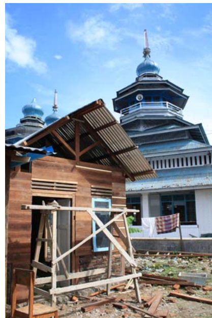
Beneficiaries in West Sumatra can now opt to build rumah tumbuh , a modified T-shelter that offers more flexibility in its construction and use. (Photo by IFRC/Helena Rea).
