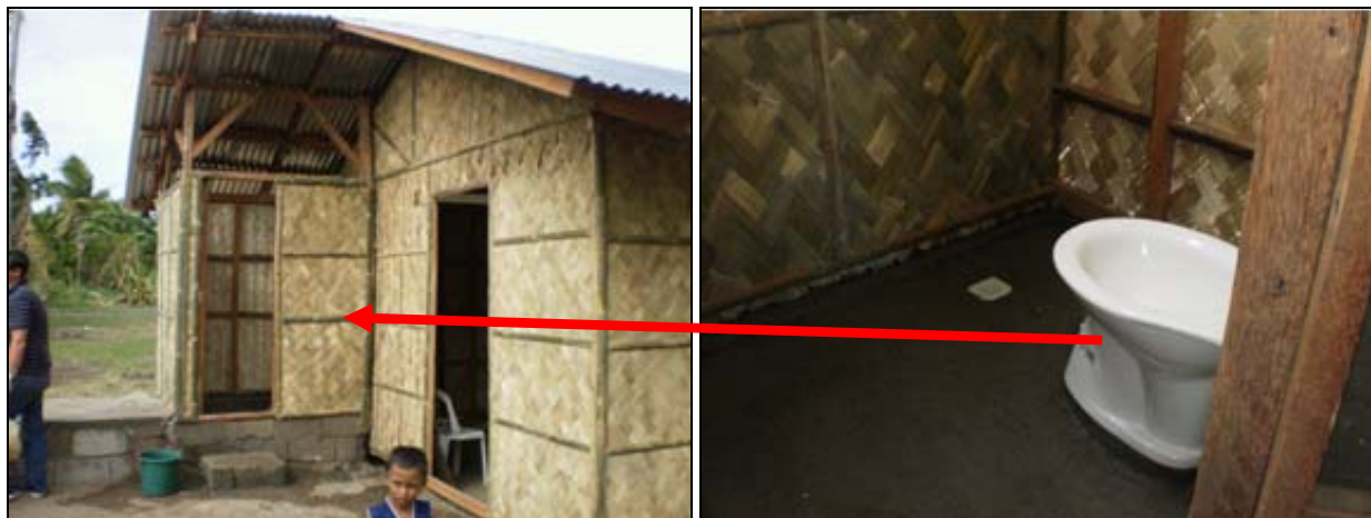
A pour-flush latrine is planned for each transitional shelter. Photo: Philippine Red Cross
