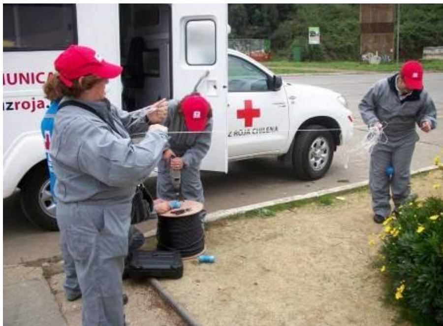
Volunteers in the telecommunications course, installing equipment in the field, in the district of San Pedro de la Paz, Bio Bio region. Source: CRCh.
