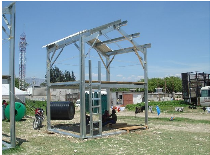
Example of the IFRC prototype of transitional shelter (urban model). Source: Hope Weiner/ IFRC
