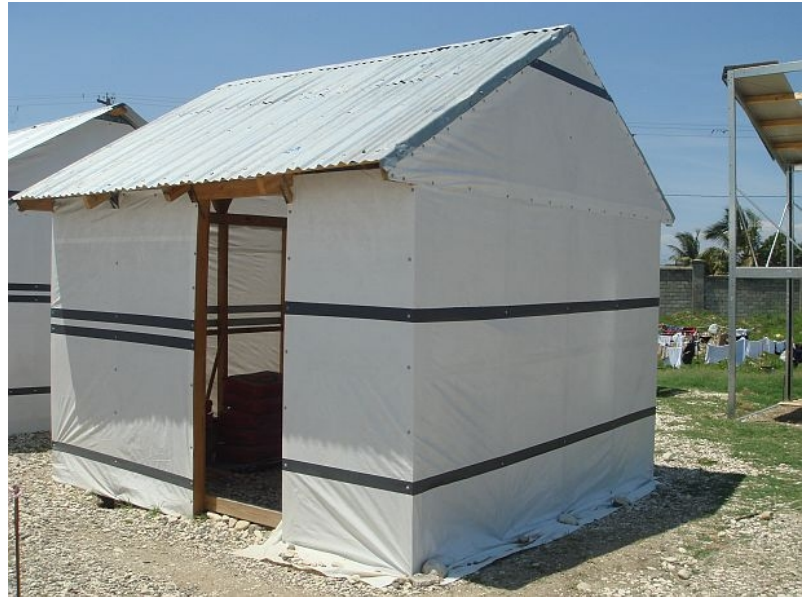
The IFRC shelter team is working on developing designs for shelter. Above, an example for the core shelter prototype. Source: IFRC
