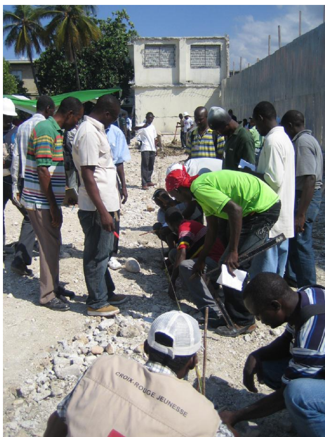
Volunteers from the Haitian National Red Cross Society participated in a training for carpenters, supported by the Canadian Red Cross in Jacmel. Source: Canadian Red Cross
