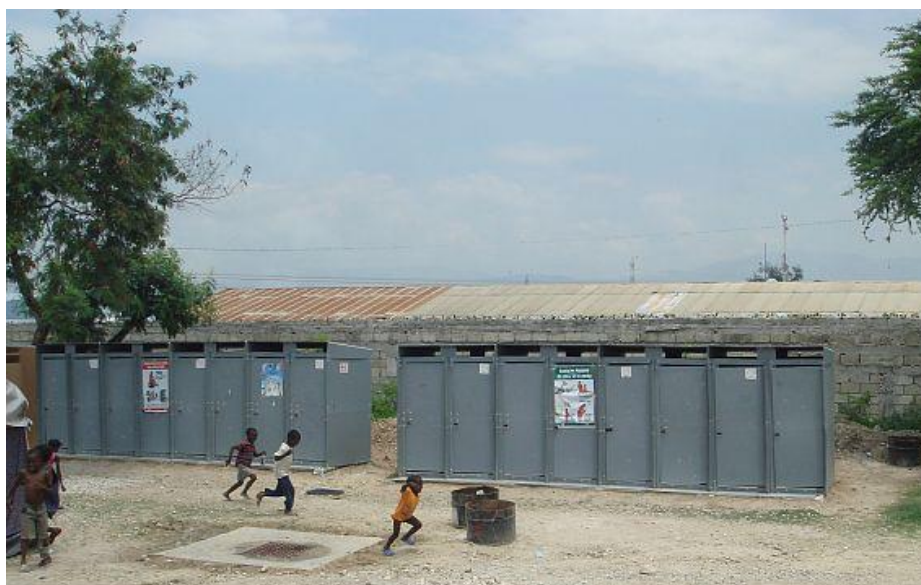
Haitian children play in the Automeca settlement. In the background, prefabricated tank latrines have been installed by the British Red Cross Sanitation ERU. Source: International Federation
