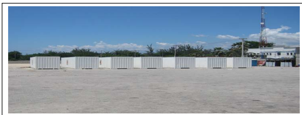
TMSUs in Barbancourt warehouse (Port-au-Prince)
