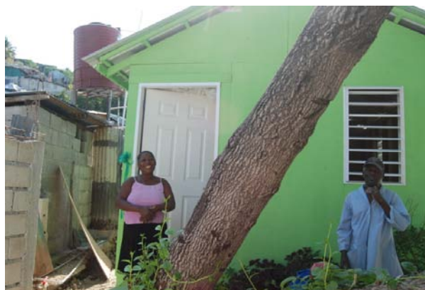
Marie Vixmant and her father in law. Marie returned to her plot of land in mid-2010, cleared the rubble and constructed a small house Source: IFRC
