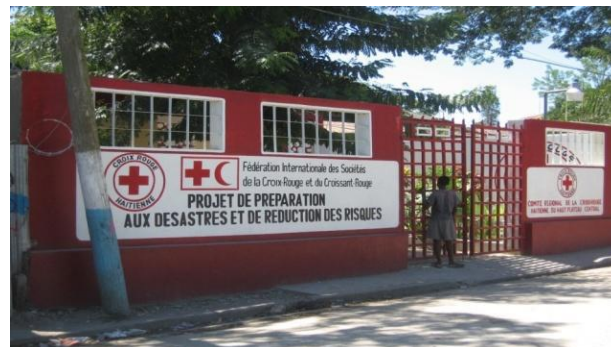
The Disaster Management Operations Centre in Hinche. Source: IFRC
