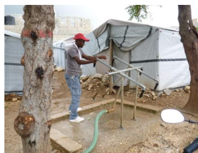
Repairs being done to tank stand and water stands in Port au Prince Source: IFRC
