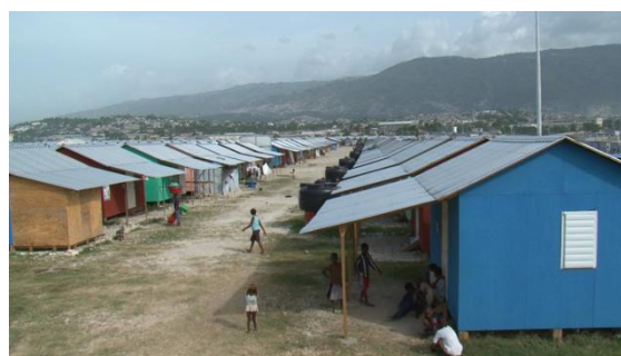
Transitional shelter units constructed at La Piste Source: IFRC
