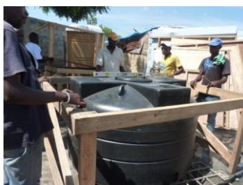
Tank latrine under construction Source: IFRC
