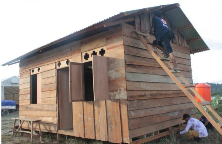
PMI volunteers work with one of the shelter beneficiaries. This shelter is almost complete, using good island timber. Wooden walls are expected to withstand the extreme weather currently being experienced on the island. (Photo: Palang Merah Indonesia).
