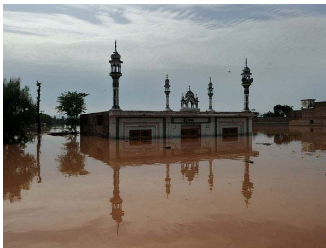
A mosque half submerged in water during the recent floods. The flood water rose in Swat (Khyber Pakhtoonkhwa) seven to ten feet high, damaging the houses, schools and other infrastructures. Photo: Pakistan Red Crescent Society communication.
