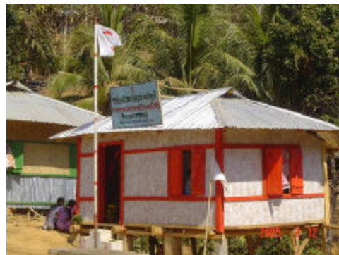
Chittagong Hill Tract development programme field office constructed by the community on their own initiative.
