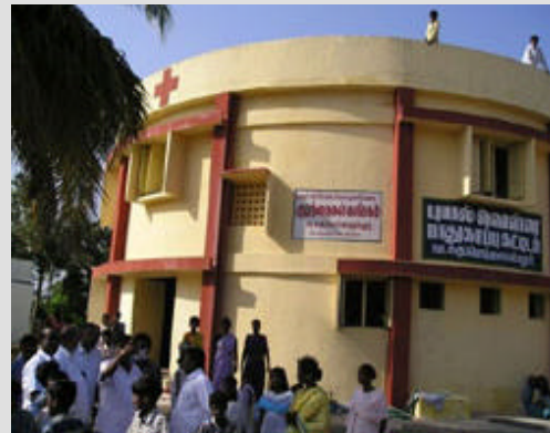
An Indian Red Cross cyclone shelter in Tamil Nadu, built as part of the disaster preparedness programme, is now used as a relief centre following the 26 December tsunami.
