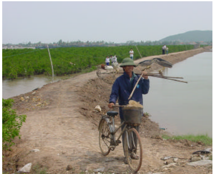
No dyke was broken or damaged during the Typhoon Damrey thanks to mangroves planted by VNRC in 1997.
