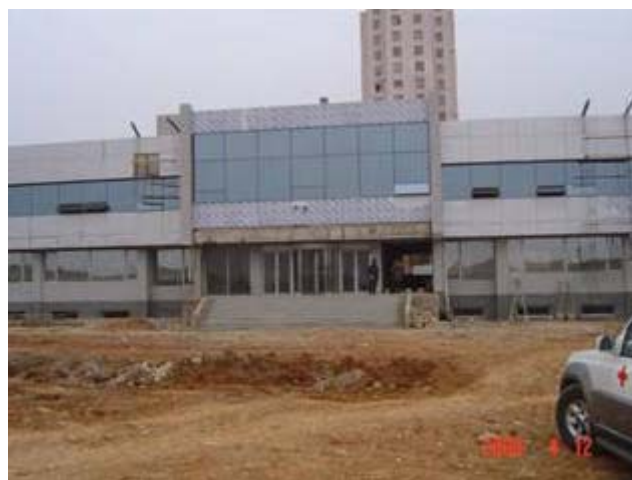
Work in progress on the Red Cross Pyongyang Service Centre
