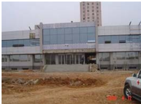
Work in progress on the Pyongyang Service Centre.
