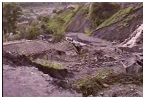
Landslide resulting from torrential rain in Sinyang County (South Phyongan province)
